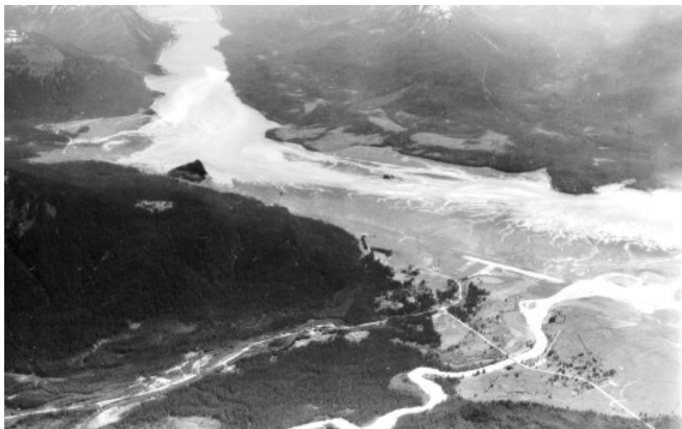
Oblique View Over the Incipient Juneau Airport in About 1934
